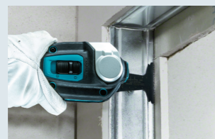
Door opening work
