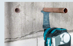
Copper pipe flush cutting
