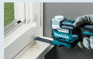
Removal of window frame
