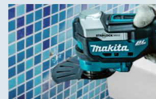
Routing joints on wall tiles
